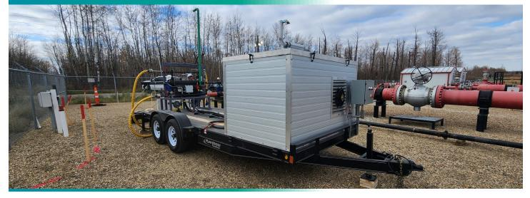
CHZero Emissions offers Zero-Flare pipeline, vessel and oilwell blowdown capture services to the Oil & Gas utility, production, midstream, and transportation sectors. CHZero's crew arrives on site, executes the operation, and can follow up with a report of the emissions reduced compared to conventional blowdown practices.
